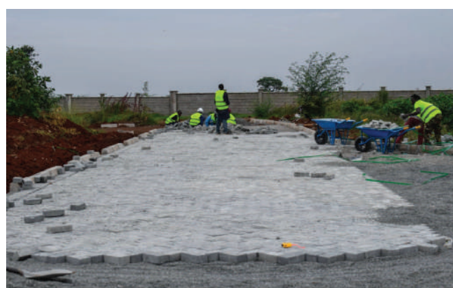
Figure 8: Internal Cabro works ongoing
