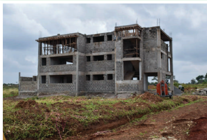
Figure 7: Club house gaining shape
